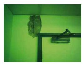
The lintel above the storeroom door extended approximately 2 inches past the edge of the recently installed doorset. Current regulations state a minimum 4 inches must protrude beyond the doorset into the brickwork on each side. The lintel did not appear to be of new construction.
