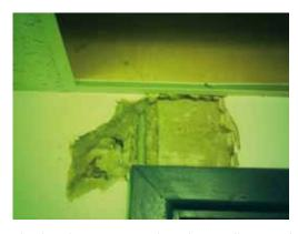
The lintel was original and actually rested on the new doorset. Current regulations state a minimum 4 inches must protrude beyond the doorset into the brickwork on each side. In addition it was noticed that there was evidence of cracking from the corner of the doorset and travelling upwards. It is not known whether this cracking was in existence prior to the new doorset and/or its structural significance.
