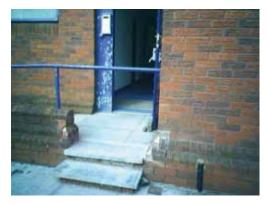
The contractor has provided two steps to the landing of the ramp. It is not known why the provision of steps to an existing ramp would be required under Disability Discrimination legislation. The existing handrail was not modified to permit the use of the steps thus creating a hazard in the event of an emergency.
