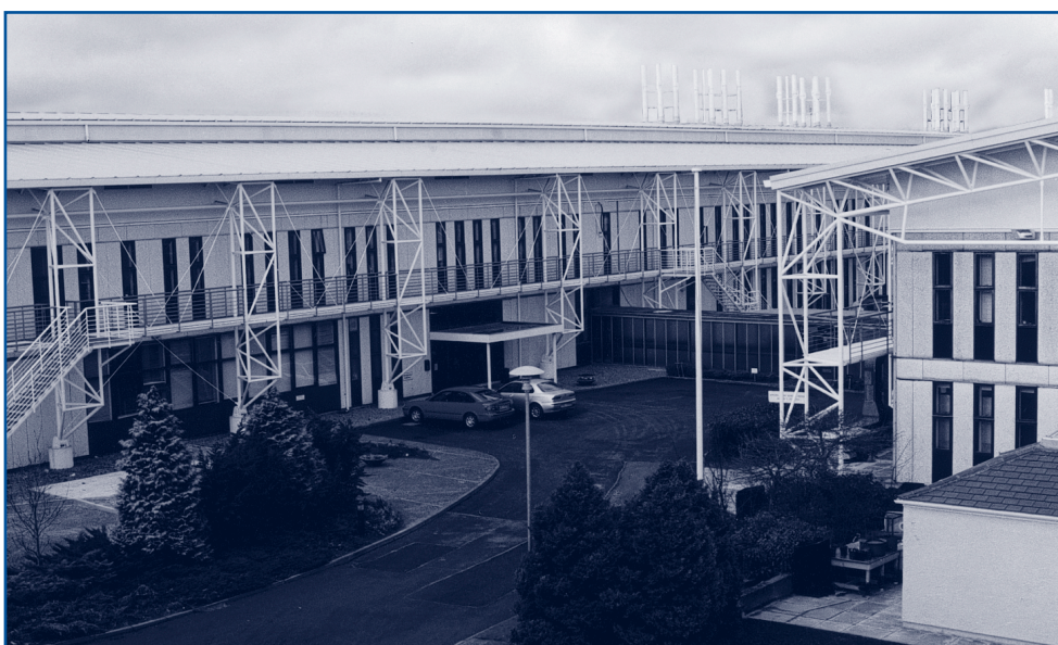
Re-roofed blocks at the Centre
