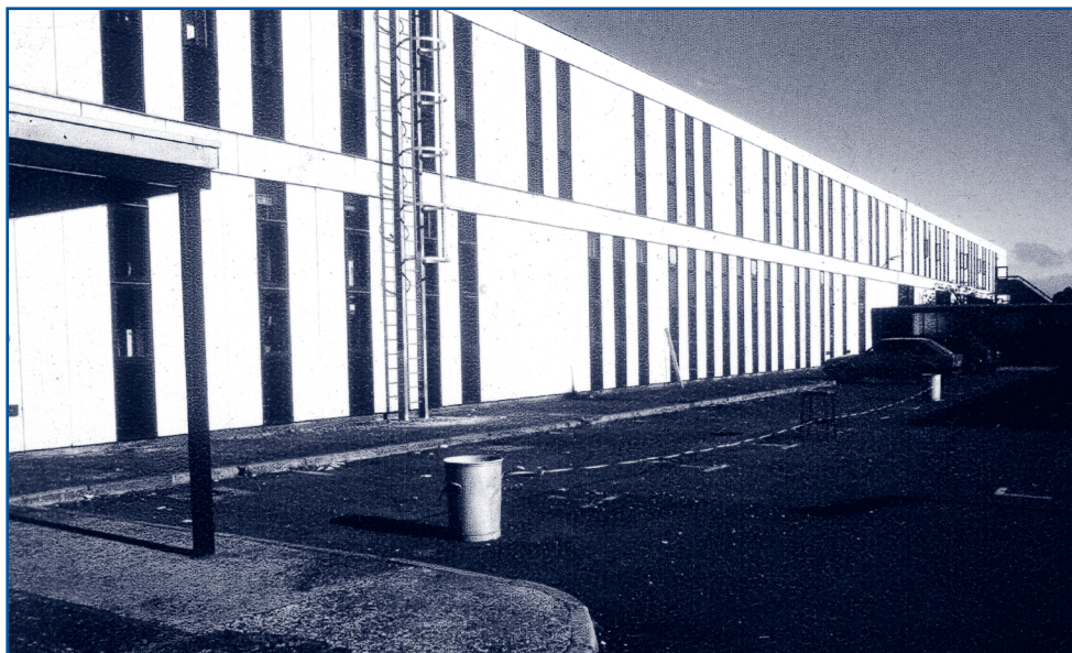
Flat roofed block at the Centre before re-roofing
