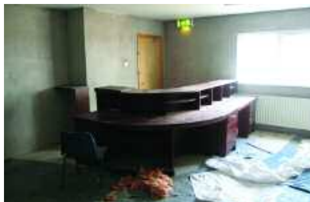
Unfinished reception area.
