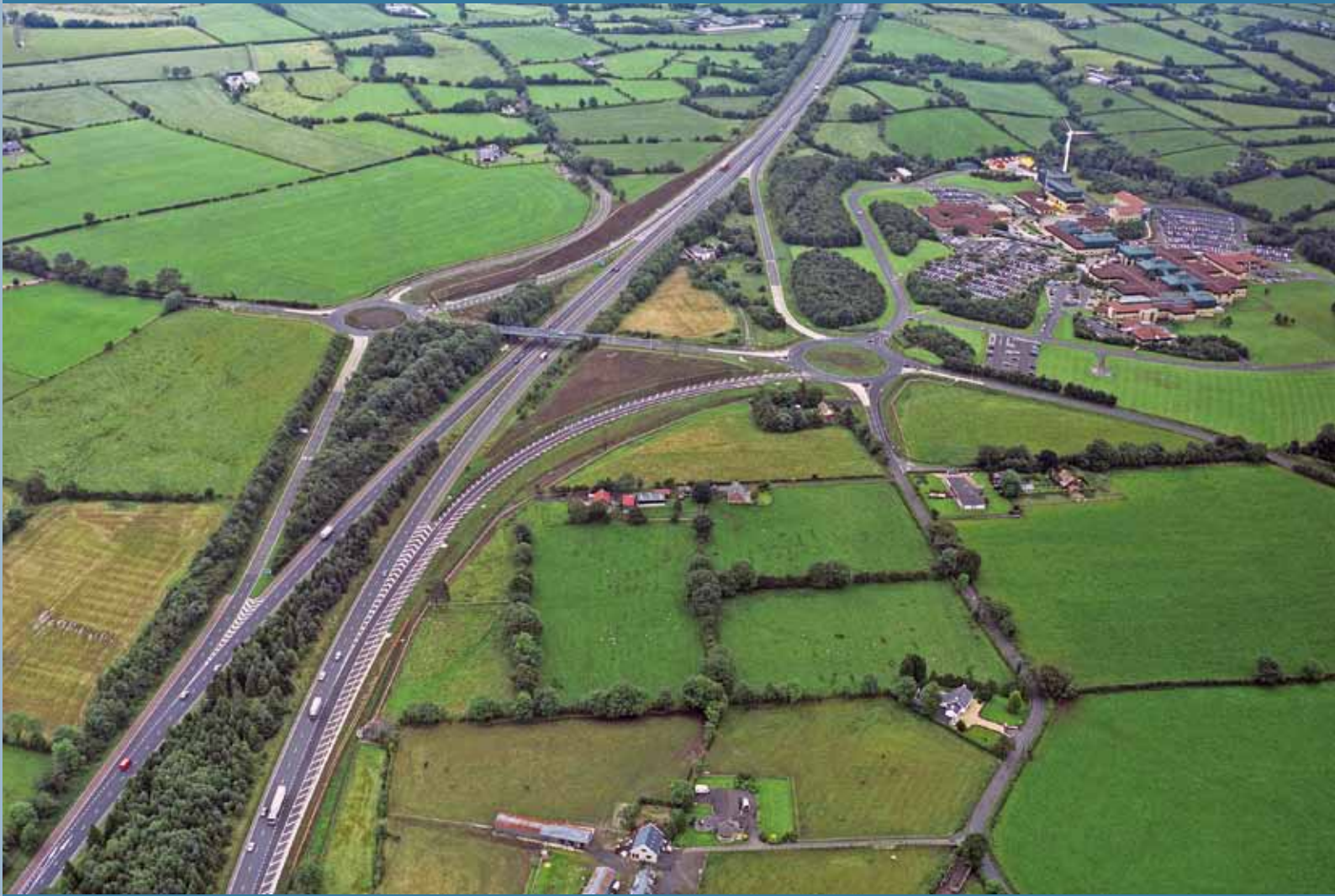
M2 Antrim Area Hospital slip roads
