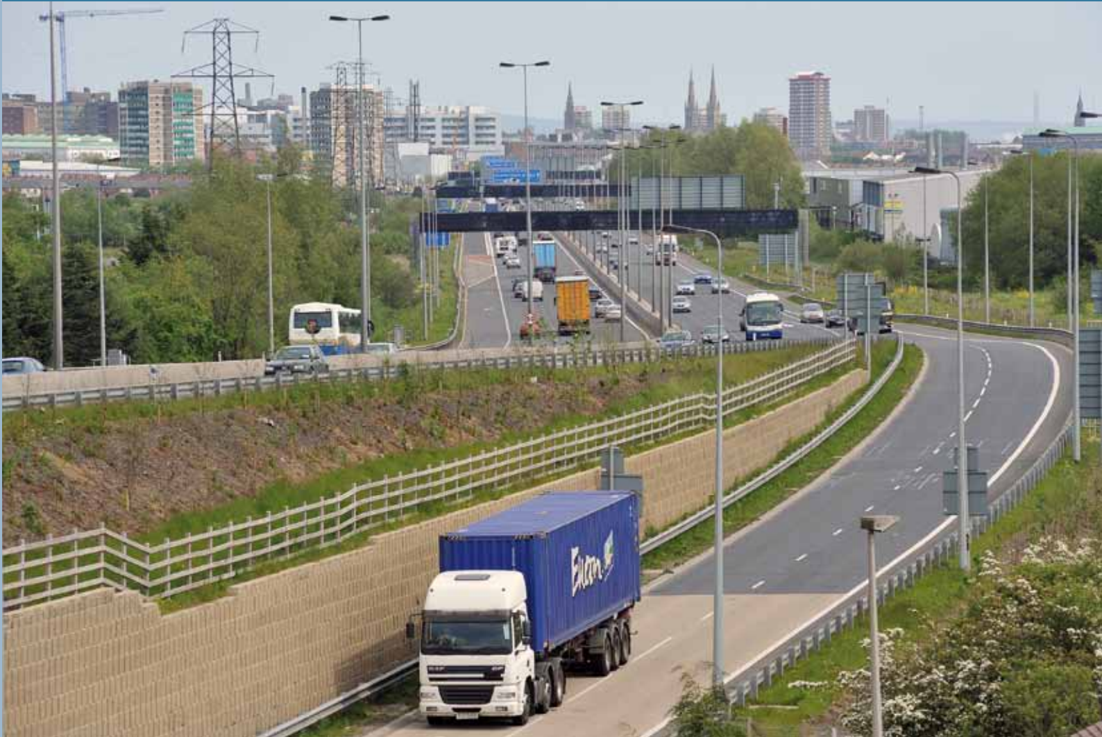
Westlink road improvements
