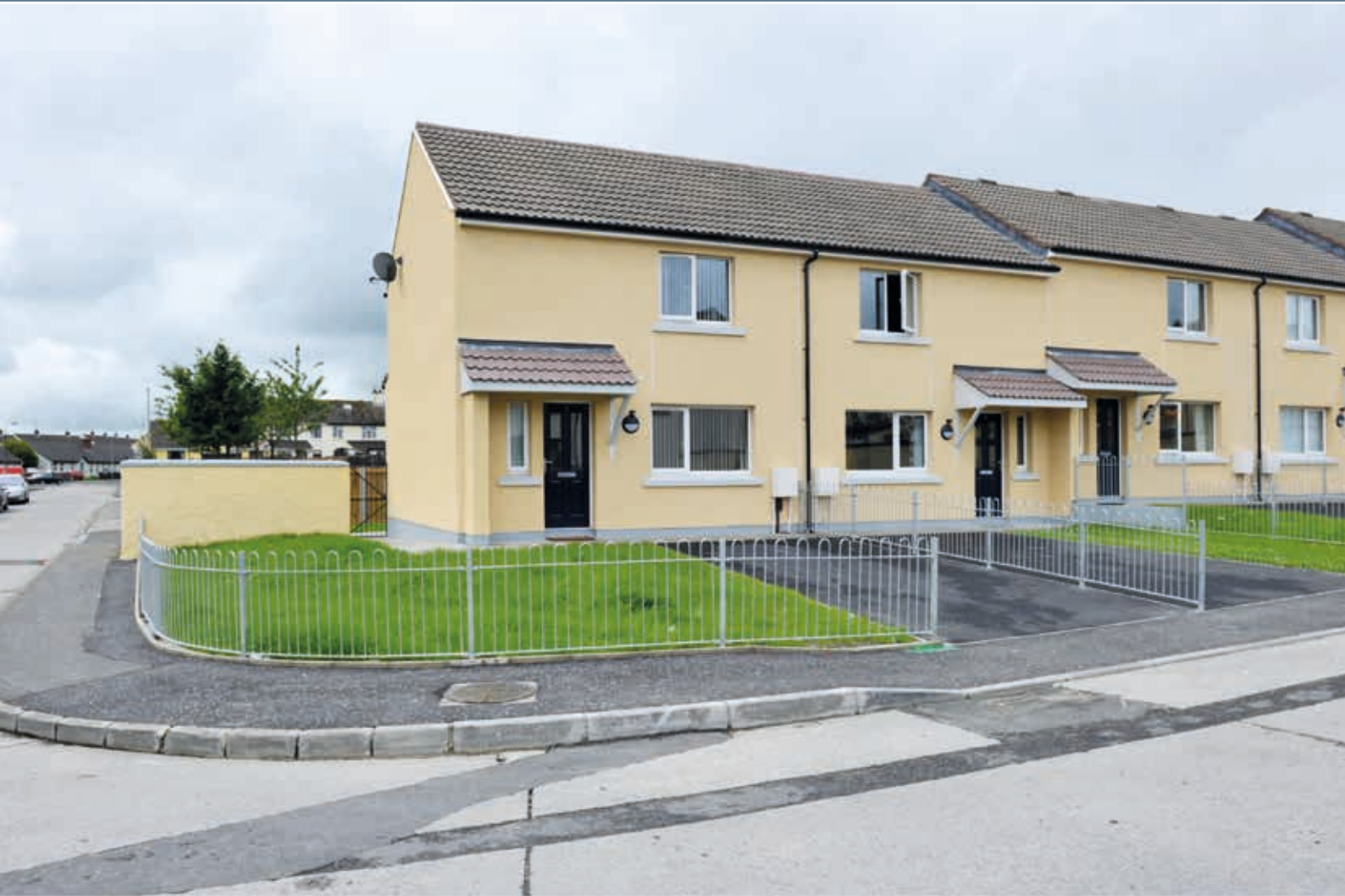
Houses at Rinmore after refurbishment: photo courtesy of DSD
